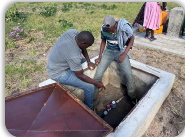
LEFT: Accessible pipes near a water distribution point for easy maintenance.
